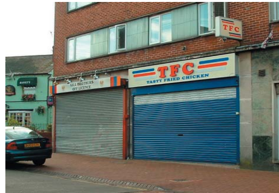
Fig. 57. Example of poor roller shutter design that impinges on window shopping and creates an unattractive shop frontage.
