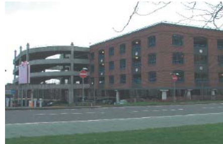
Fig. 74. Park Mark® car park, Telford
