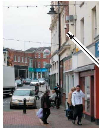
Fig. 72. CCTV discreetly positioned on the wall of a building. Wellington Town Centre.
