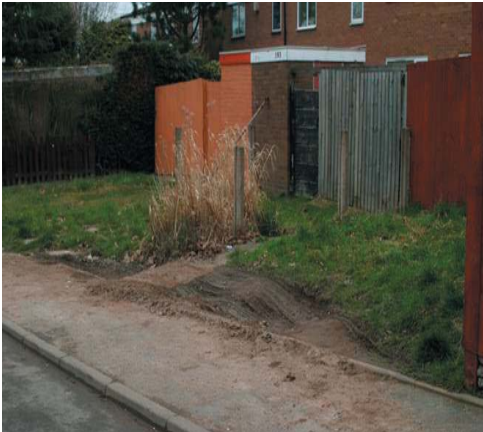
Fig. 19. A Telford estate where private and public space is not clearly defined leading to poor sense of ownership and increased vandalism and crime.
