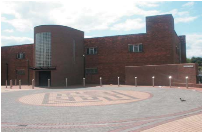
Fig. 88. Well maintained area - simple bold design using good quality materials.
