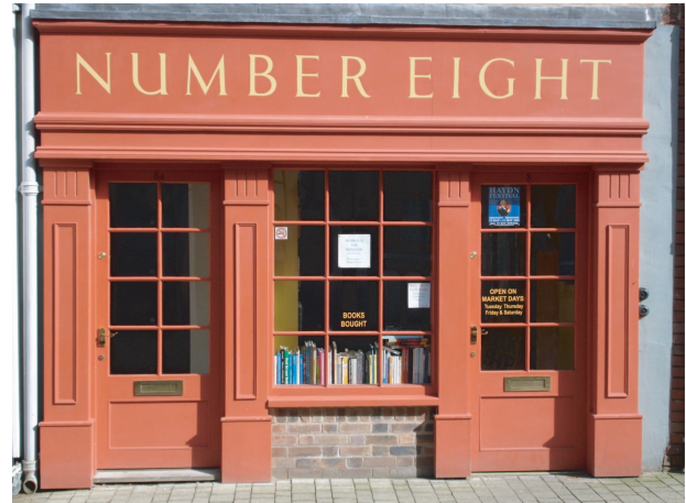
Picture 13 GOOD : Fascia
