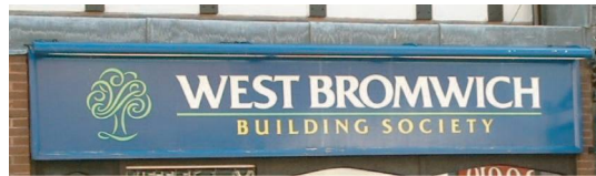
Picture 25 GOOD : Unobtrusive trough lighting running along the top of the sign board
