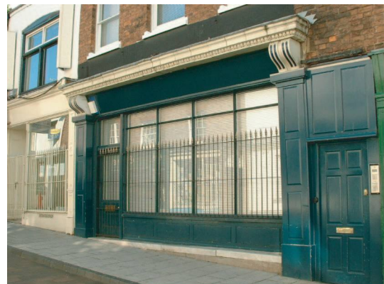
Picture 27 GOOD : Use of demountable decorative ironworks presents a much more appropriate frontage within a Conservation Area than roller shutters
