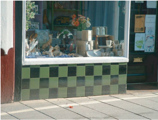
Picture 2 GOOD : A good example of a decorated stall riser, mid-late 20th century contrasting glazed tiles are used to good effect
