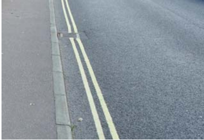
5a. Drainage channel within blacktop road
