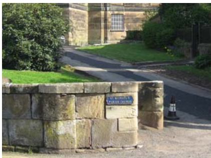
I4a Ashlar stone boundary wall
