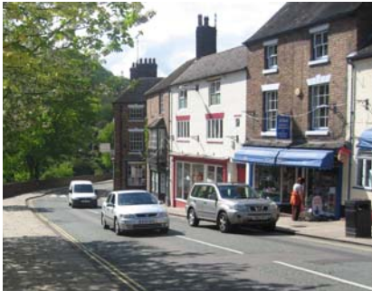
9a. Wall mounted street lighting
