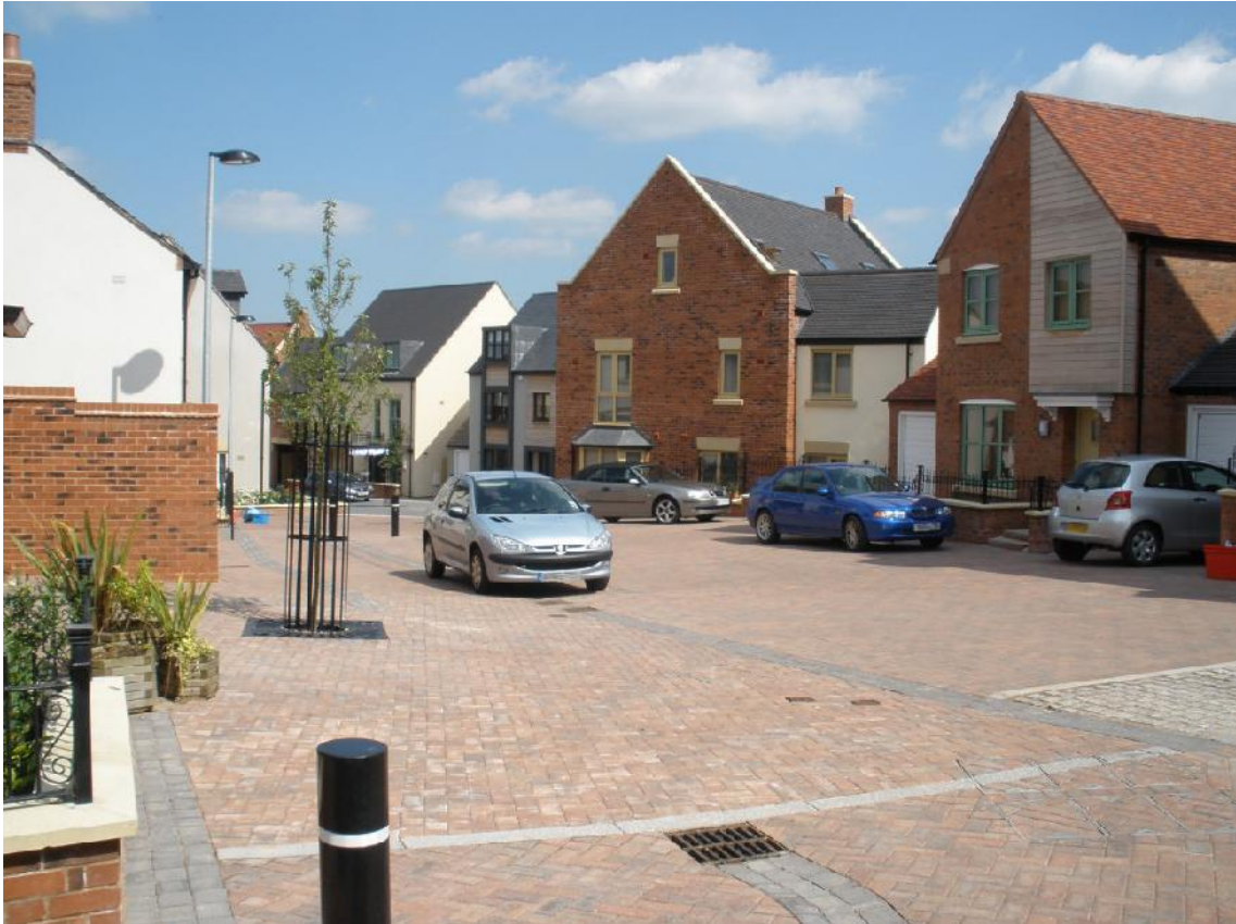
Picture 8 Housing - St Johns Walk, Lawley, Telford
