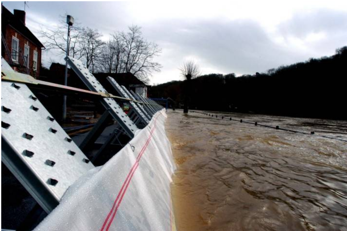
Picture 14 Flood Defences - Ironbridge, Telford
