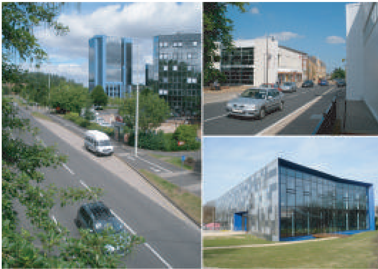
Picture 3 The Borough's Economic Offer - Telford Town Centre, Madeley and Hortonwood.
