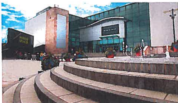
Picture 4.1 Retail in Telford Town Centre
