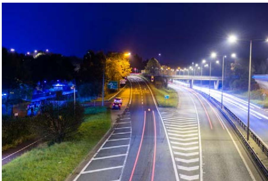
Picture 33 A442/Queensway/Eastern Primary through Telford
