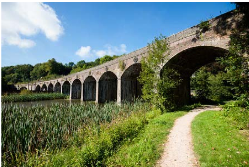
Picture 4 Coalbrookdale Viaduct, Coalbrookdale, Telford.
