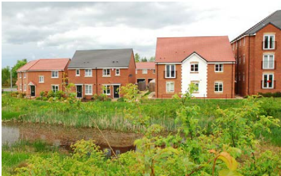
Picture 23 Multifunctional green infrastructure providing amenity, biodiversity and SUDs
