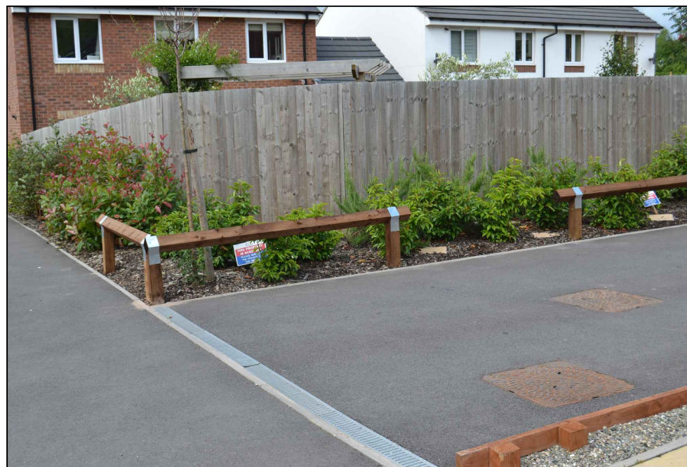
Photo of Diamond Rail barrier rair to rear of 7 Cloisters Way.
