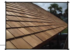
CEDAR SHINGLE ROOF
