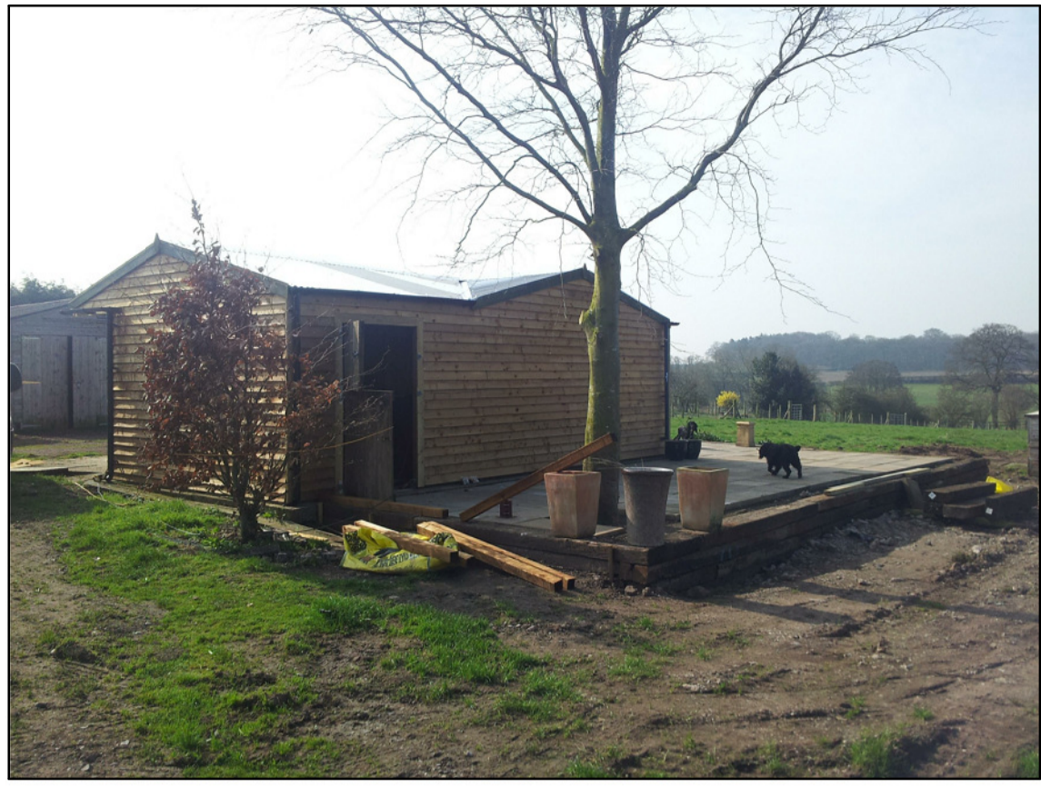
View of Existing shower block
