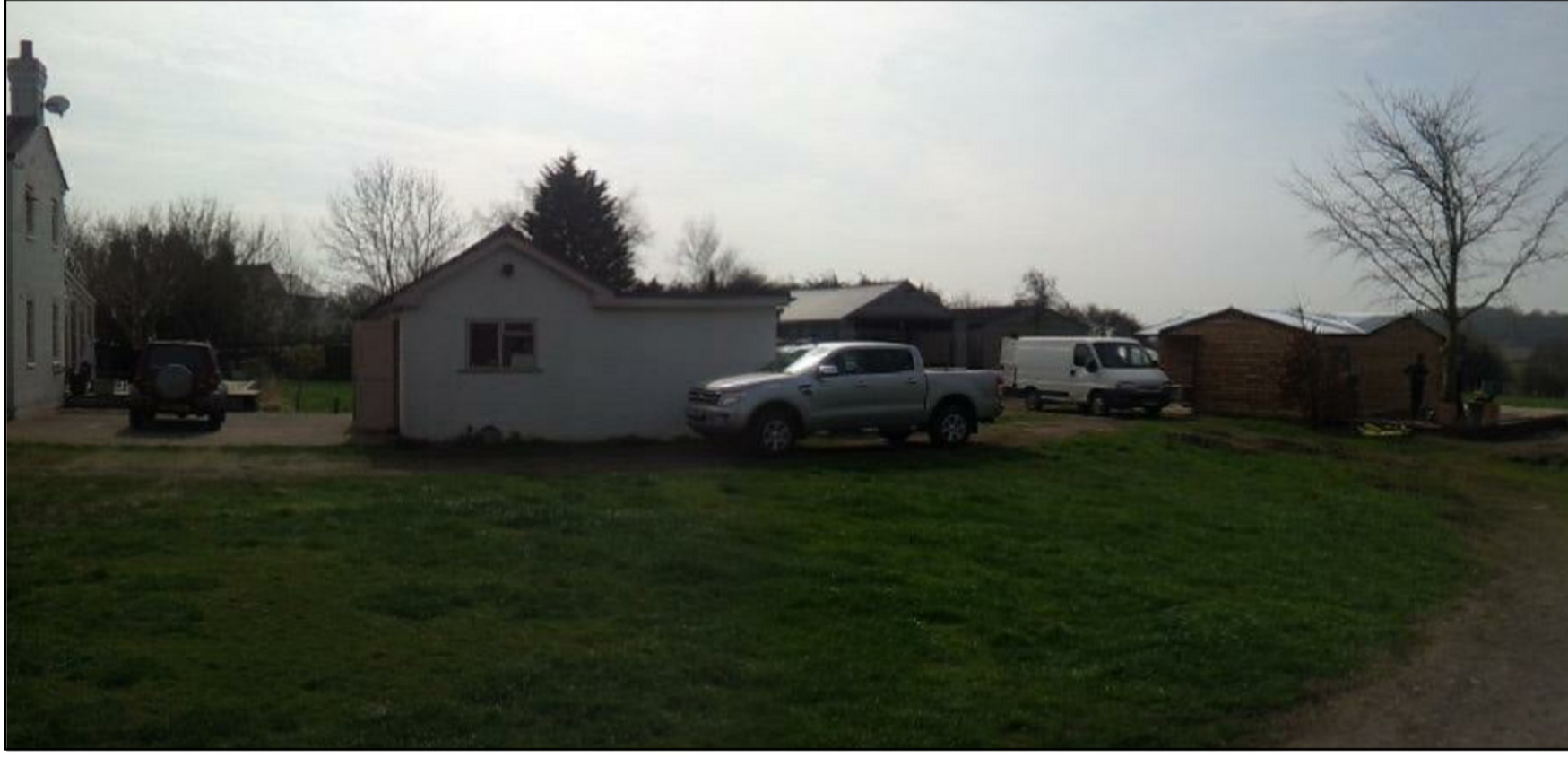
View of separation between Existing shower block and Store
