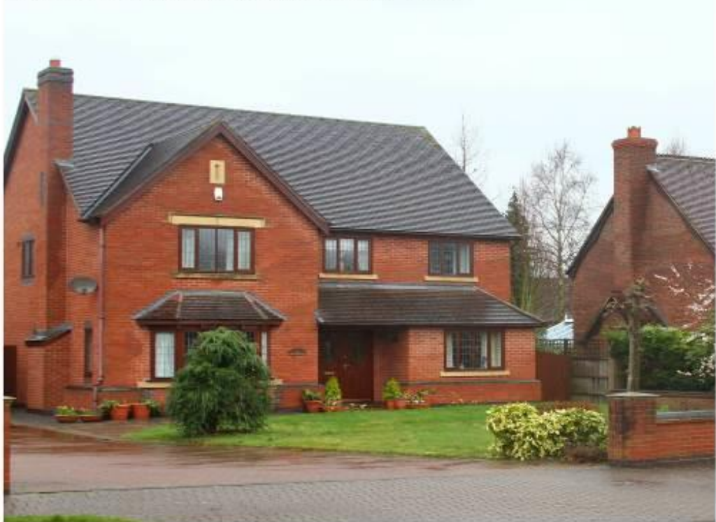
existing house - Peregrine Way
