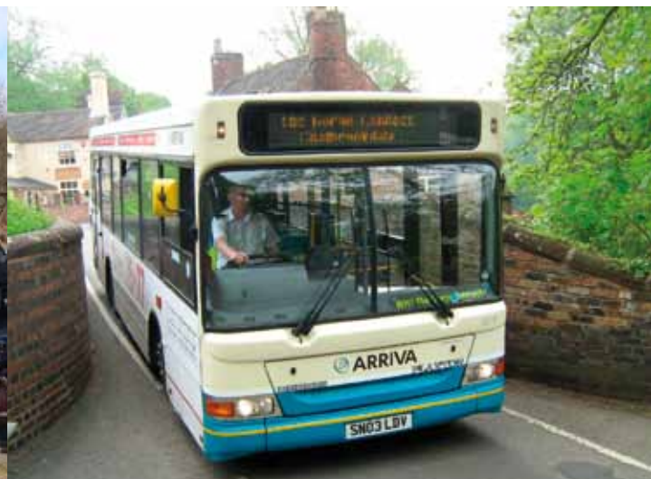
Narrow bridge over the Hay Inclined Plane in Coalport
