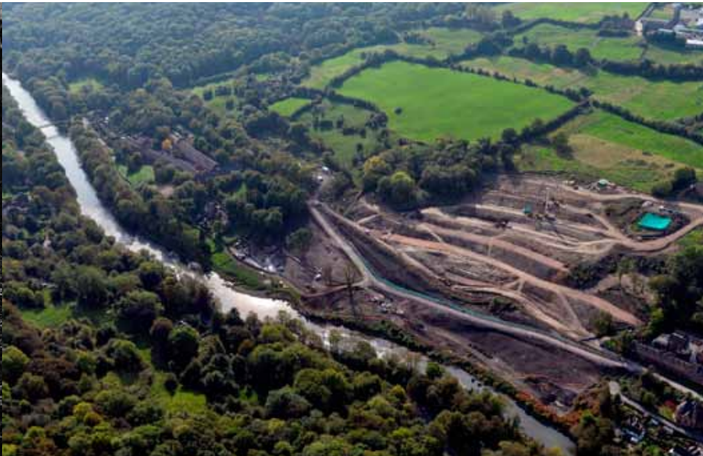
Jackfield Stabilisation Project
