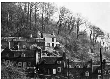
Pan Shop Bank, Coalbrookdale, c.1952
