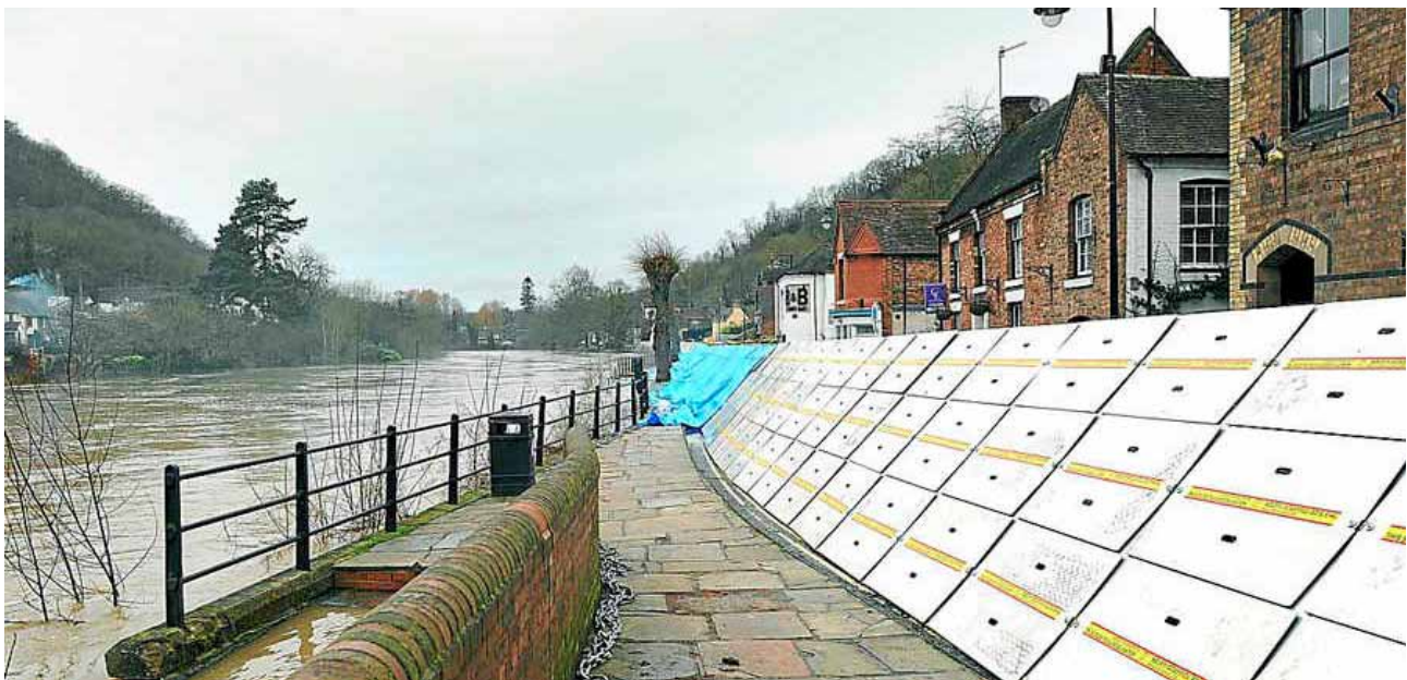
Ironbridge flood barriers
