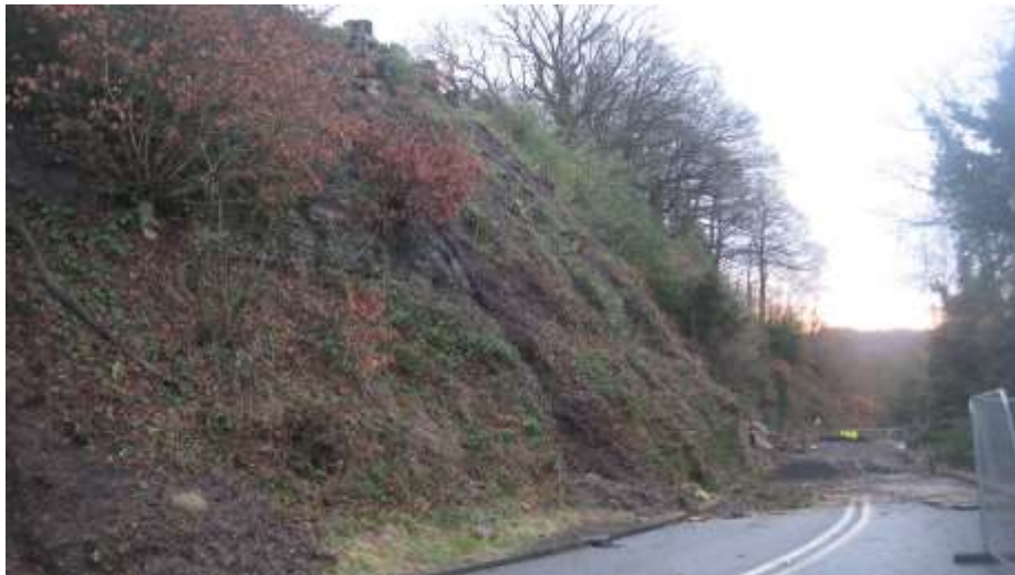
Carriageway and Footway
