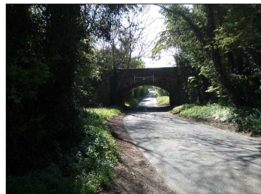
View towards Red House Inn Roundabout
