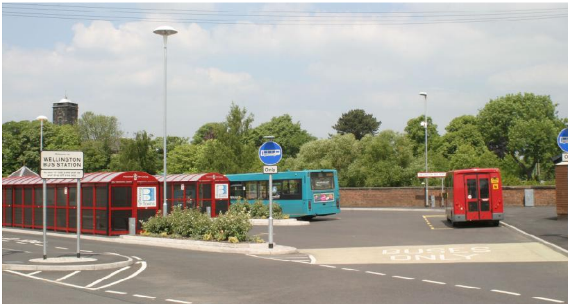
Picture 10 Wellington Bus Station, Telford
