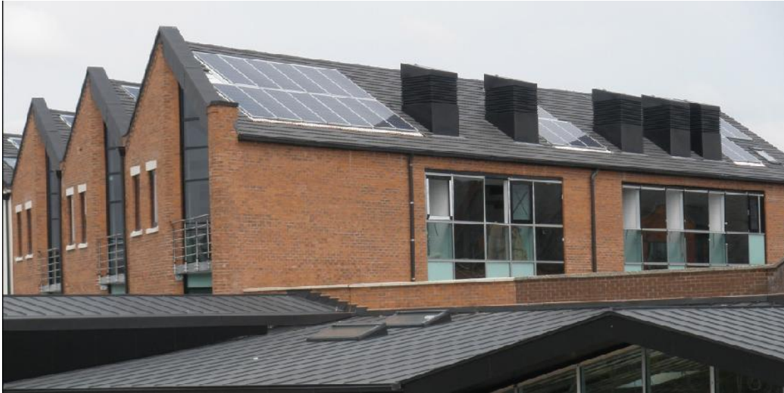
Picture 13 Renewable Energy - Wellington Civic, Telford
