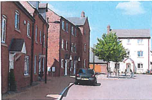
Picture 3.1 Recent development in Horsehay, Telford
