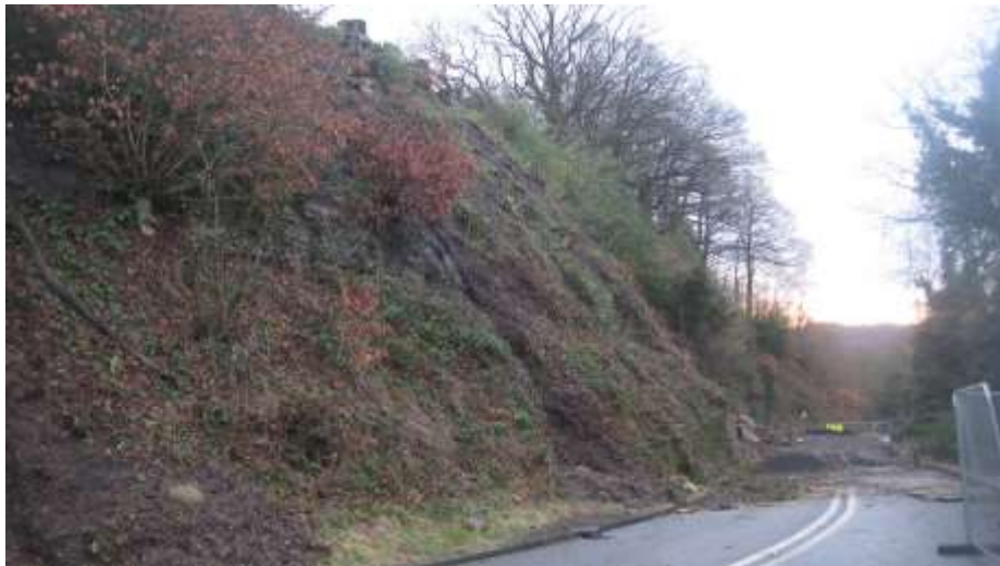
Carriageway and Footway
