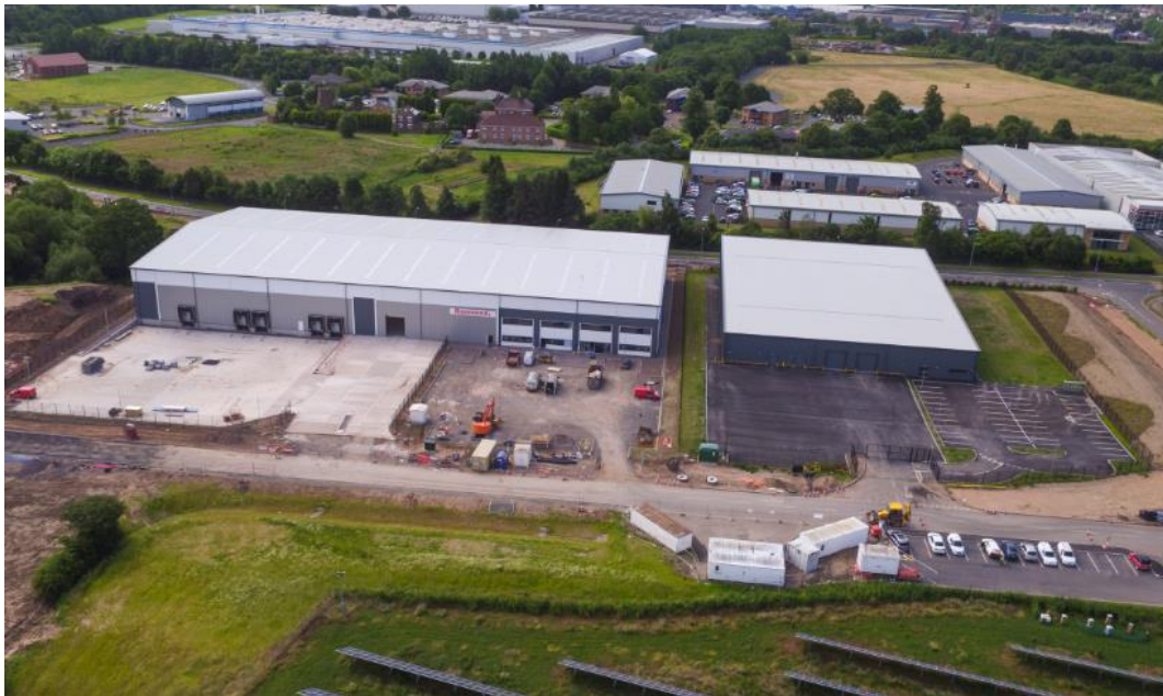
Units 9 & 10 Hortonwood West – June 17
