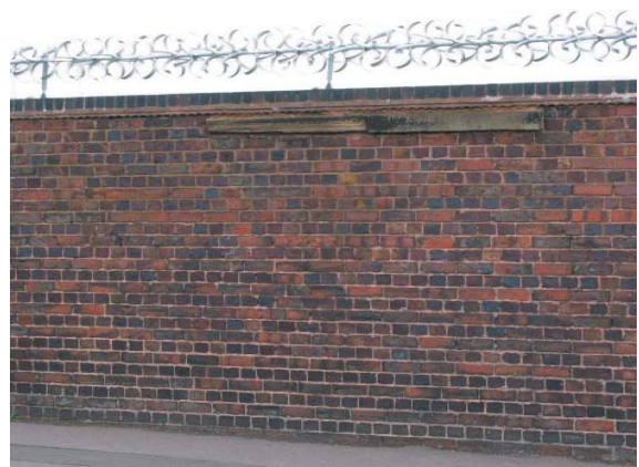
Fig. 33. Cacti anti-scaling device to be used in high risk areas only
