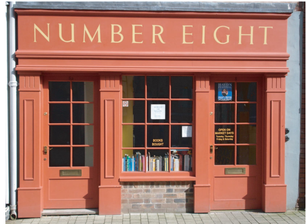
Picture 13 GOOD : Fascia
