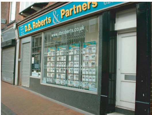
Picture 26 GOOD : Use of internal grilles on this modern shop front allows shop security to be maintained whilst allowing window shopping and advertising to continue out of hours, it provides a much better street impact that the shuttered property next door
