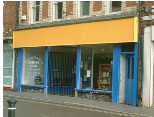
Picture 15 POOR : Oversized boxed out fascia board with no cornice or architrave or capitals to enclose it or support it. It dominates the shop front to an oppressive degree
