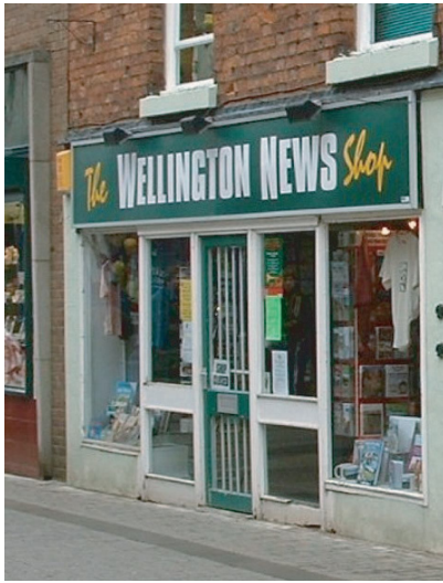
Picture 18 BEFORE : Door and signage
