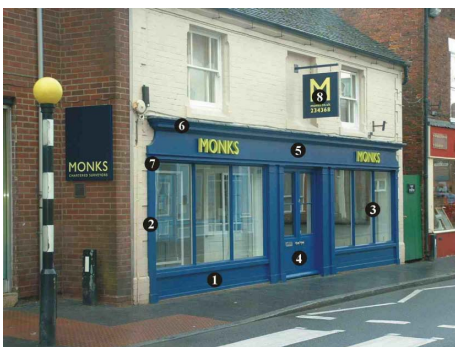
Picture 9 GOOD : Example of simple mullions used to reduce a large area of glass
