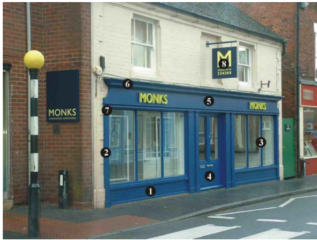
Picture 9 GOOD : Example of simple mullions used to reduce a large area of glass
