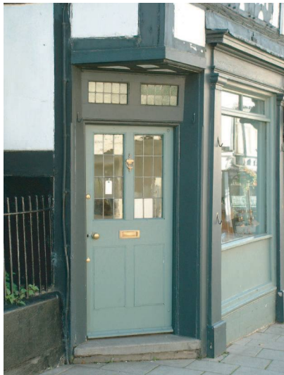
Picture 16 GOOD : Leaded glazed panels to upper lights picking up fanlight details
