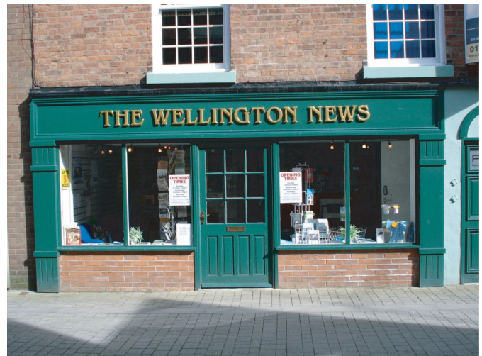
Picture 19 AFTER : Door and signage
