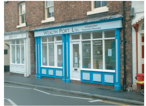
Picture 10 GOOD : Example of the use of high level transom to create to allow ventilation
