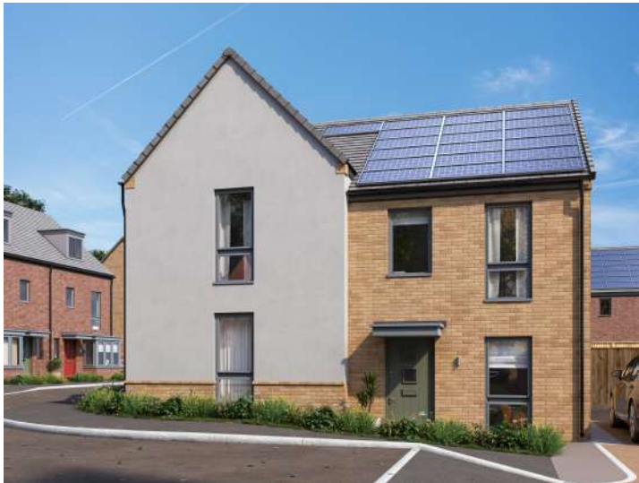
Figure 14: Solar panels on Residential House
